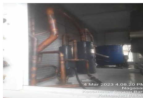
Figure 7. Freezing disappears after adjustment of the refrigerant mass flow rate with globe valve
