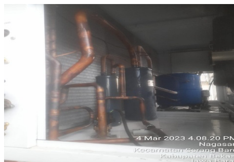
Figure 7. Freezing disappears after adjustment of the refrigerant mass flow rate with globe valve
