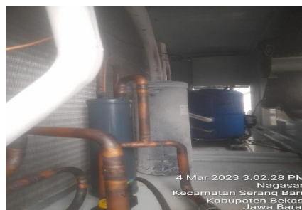
Figure 6. Freezing on gas lines
